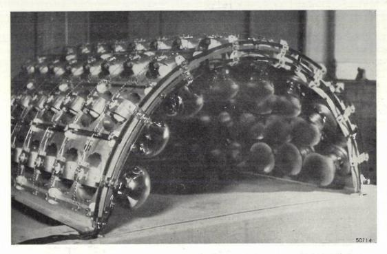
Fig. 9. A drying tunnel with Philips drying lamps, built up from "building elements" each containing one drying lamp.
