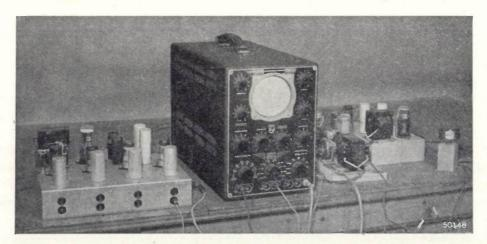
Fig. 4. Experimental arrangement of the apparatus for measuring the rate of watches. In the centre the cathode-ray oscillograph, to the left the apparatus supplying the synchronizing voltage with a frequency of 60 c/s. (see fig. 3). On the extreme right the microphone with a watch placed on top. Between the microphone and the oscillograph are shown the microphone amplifier and the apparatus for converting the ticks of the watch into voltage impulses (see fig. 1).
